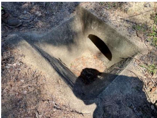
Photograph: 5 – culverts eastern end, formed at base of cutting with pipe extending across road.
