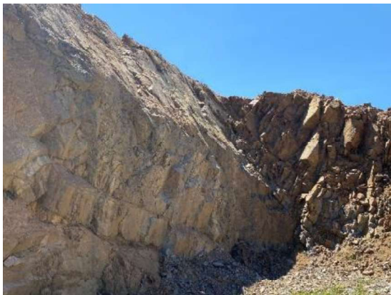
Photograph: 14 – existing quarried slope, southern end, showing continuous planar joint defects dipping east-south-east.
