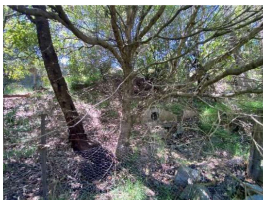
Photograph: 3 – culverts western end, formed at base of embankment.
