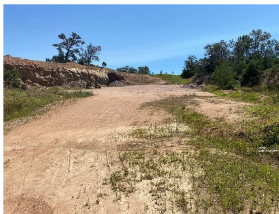
Photograph: 11 – quarry floor across eastern side, formed close to RL 152 with quarried vertical face to west and Coral Park Road to east.
