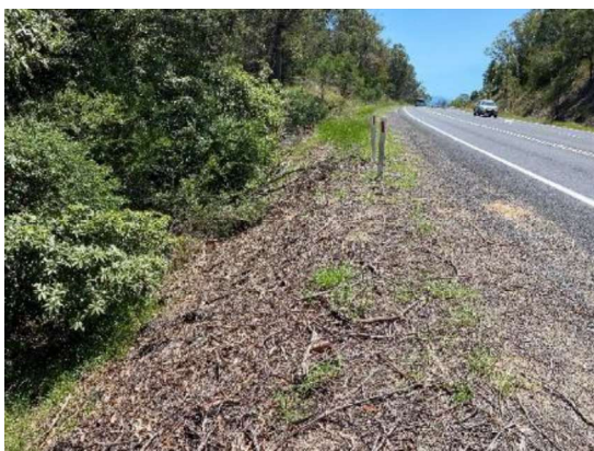
Photograph: 7 – culverts western side position, crest of road embankment.
