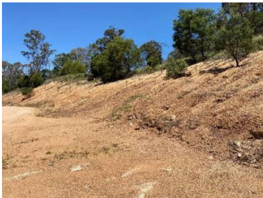
Photograph: 9 – existing batter slopes through residual soils and weathered bedrock around central to southern portion of western quarry side.
