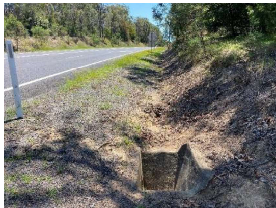
Photograph: 6 – culverts eastern end, formed at base of cutting with pipe extending across road
