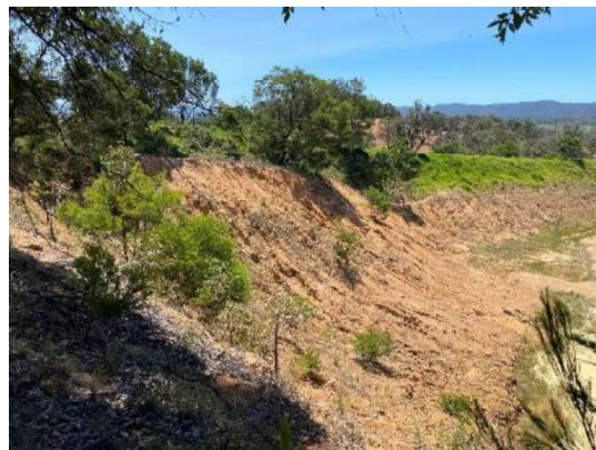
Photograph: 10 – existing batter slopes through residual soils and weathered bedrock around northern portion of western quarry side.
