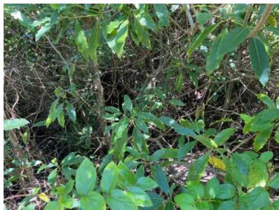
Photograph: 2 – close in view of eastern side of culvert.
