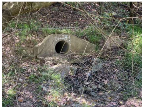
Photograph: 4 – showing exposed culvert on western side.
